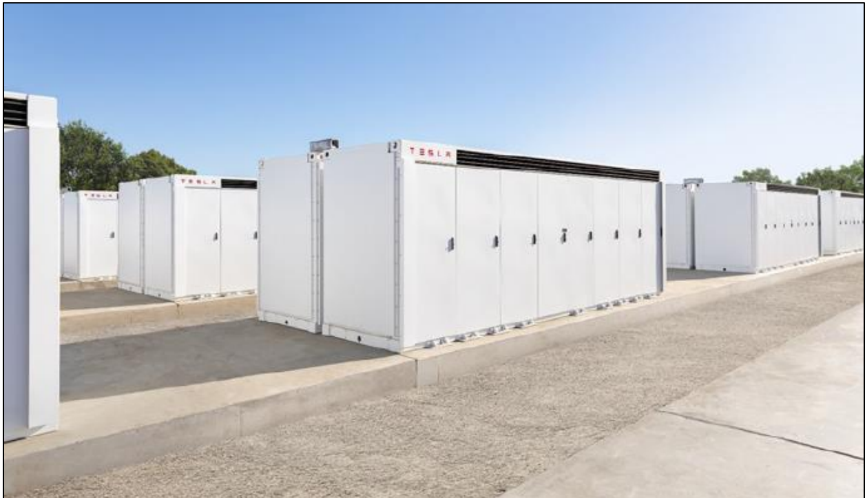
Figure 2-2 Typical Tesla Megapack Site Arrangement
