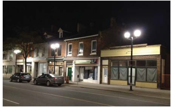
Pedestrian lighting on James Street in Hamilton provides sufficient illumination to the street, sidewalk and adjacent businesses, without need for additional facade lighting.
