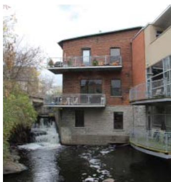
Thoburn Mill redeveloped as mixed-use building.
