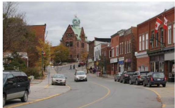
Today, the north side street wall (at left) is more porous, with many empty lots characterizing the streetscape. These lots are candidates for redevelopment.
