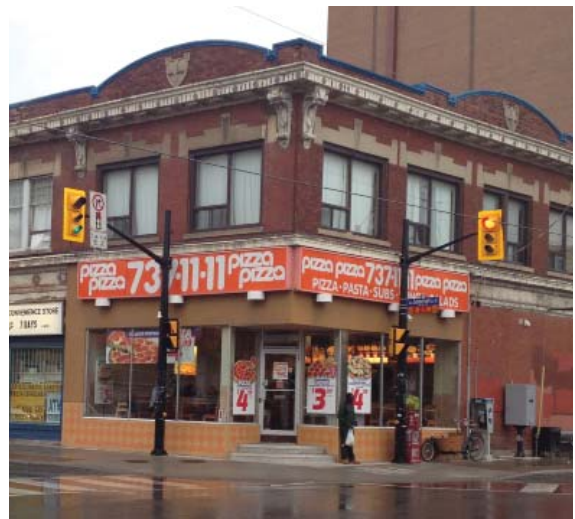
Example of a storefront alteration that is not compatible with the historic building. Original detailing has been removed and/or obscured.
