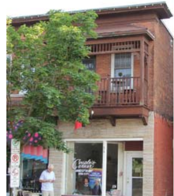
Juliet balcony on Mill Street.
