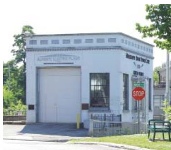
Almonte Electric Plant, an early 20th century industrial style.
