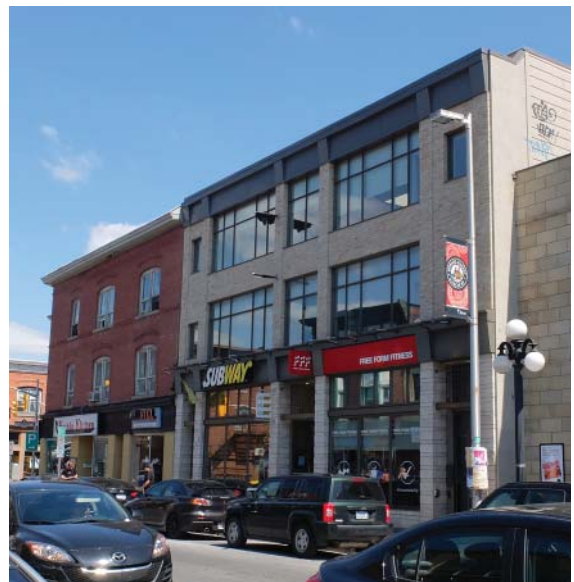
Example of contemporary infill development in downtown Ottawa that respects the rhythm and pattern of commercial facades, storefront heights and cornice lines.
