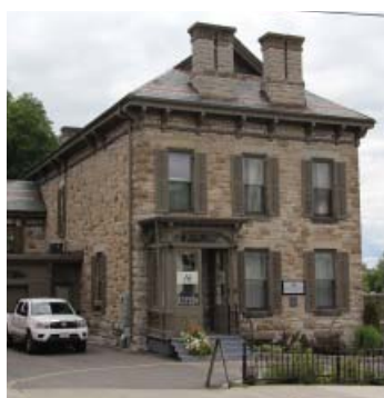
The Wylie House (aka Riverside Inn) is an example of a 'Contributing' resource whose character-defining elements have been conserved and maintained.
