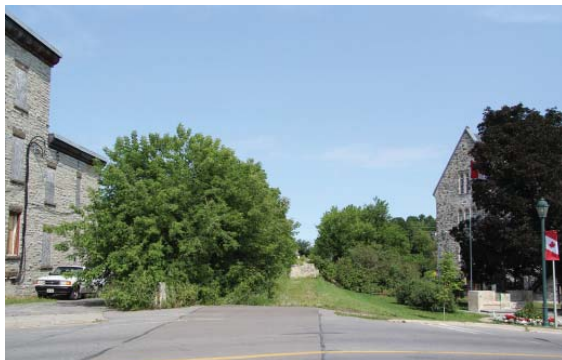
View looking north-west along the former CPR rail line at Bridge Street. Should the County acquire jurisdiction or ownership of the rail bed and bridges, it has potential to serve a recreational function.
