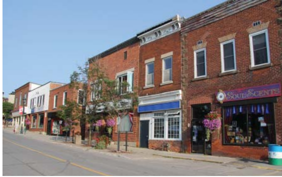
Building heights on lower Mill Street and Bridge Street are predominantly two storeys.
