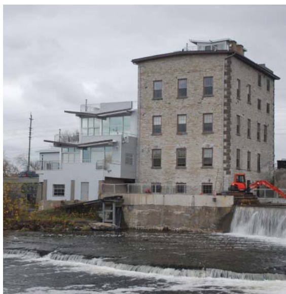
The former Wylie Flour Mill (now the Almonte Flour Mill) on Main Street East was built and operated as a grist mill. It was redeveloped as a condominium and power generating station.
