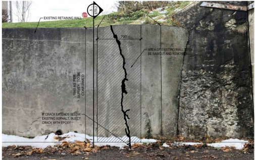
1 RETAINING WALL DEMOLITION ELEVATION STR.2 SCALE: 1/2"
