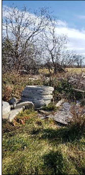
Image 3. View of the construction material located within the construction yard, facing southeast. (20201109_134915)
