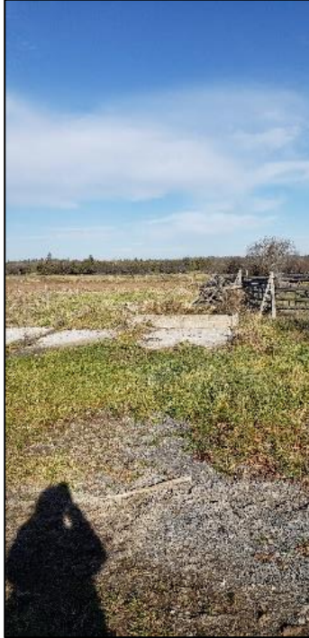
Image 7. View of the now demolished barn foundations, facing northeast. (20201109_133127)
