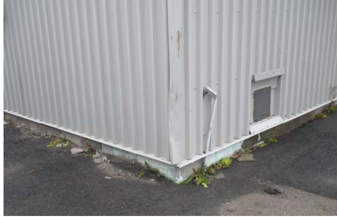
Photo 6: Well 5 - Cracked paving
