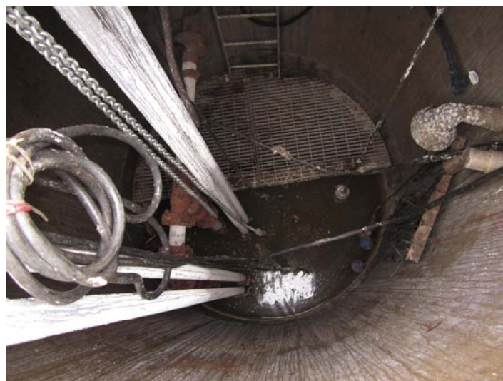
Photo 26: Robert Street SPS - Interior
