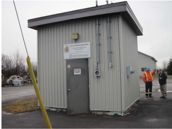
Photo 10: Well 5 - Redundant hydro meter base and conduits
