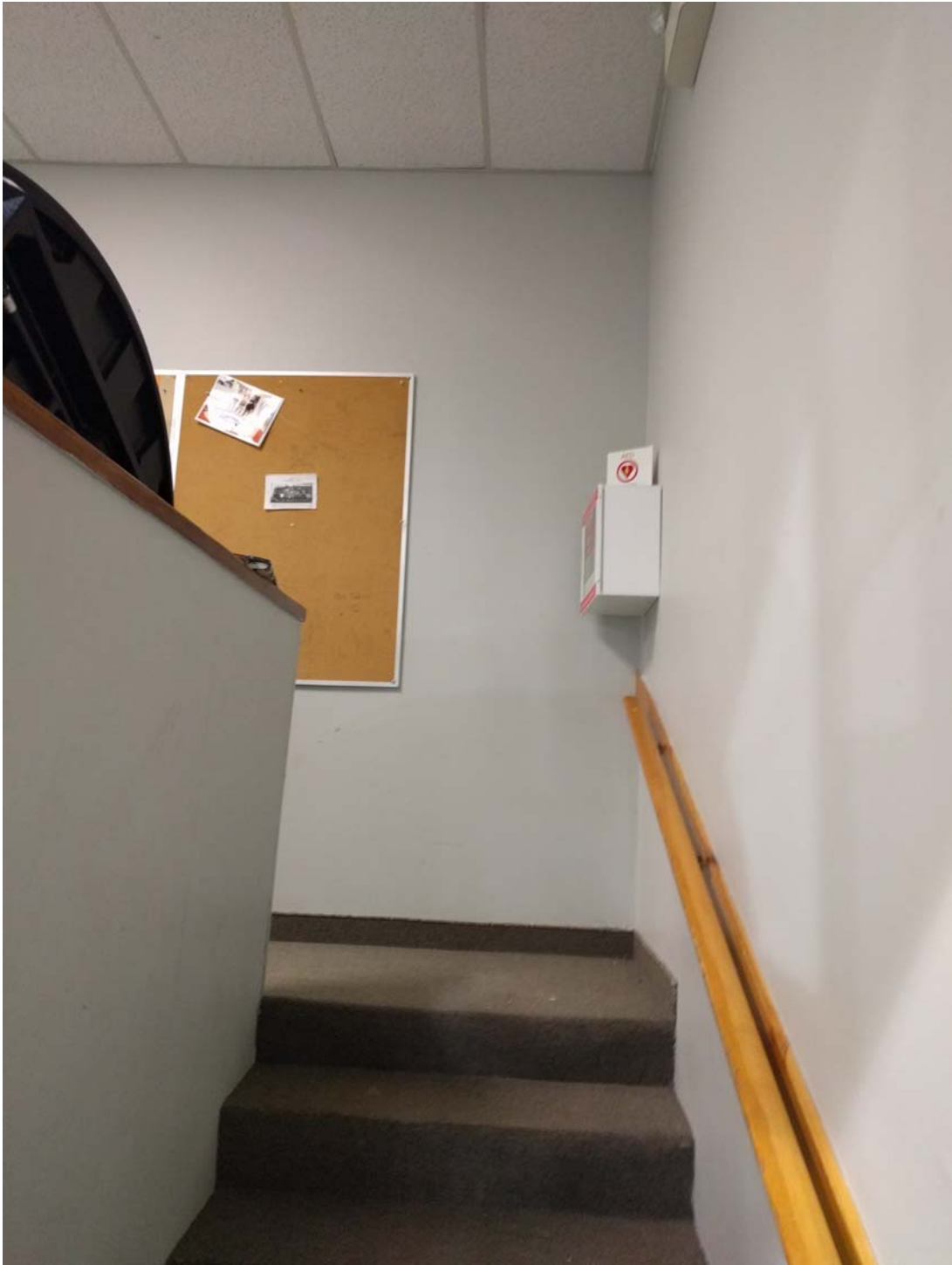
Photo 3: View from bottom landing of stairs
