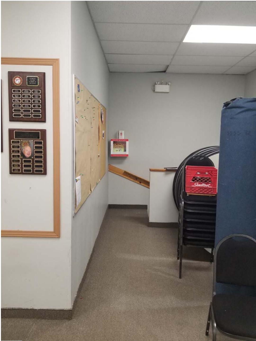
Photo 1: Upper landing of stairs in the club lounge
