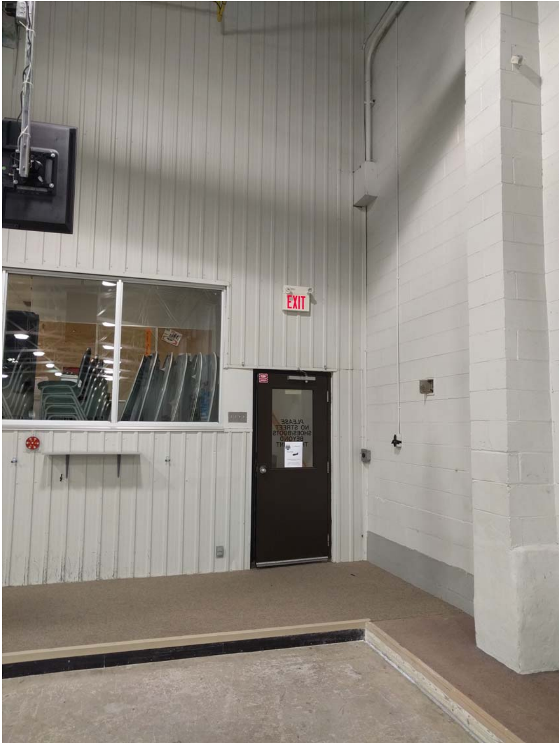
Photo 5: Doorway separating lower landing of stairs and curling rink area
