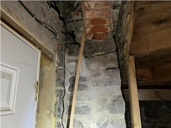
Photo 1: Separation between Inner and Outer Wythe
