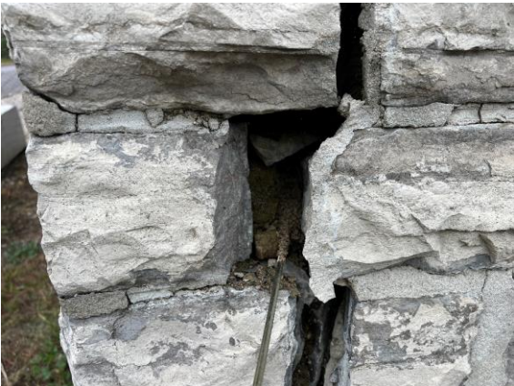
Photo 3: Core Being Raked Out
