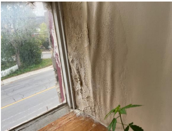
Photo 11: Moisture Damage
