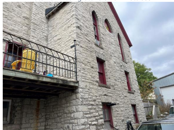
Photo 22: Representative Pointing on the East End
