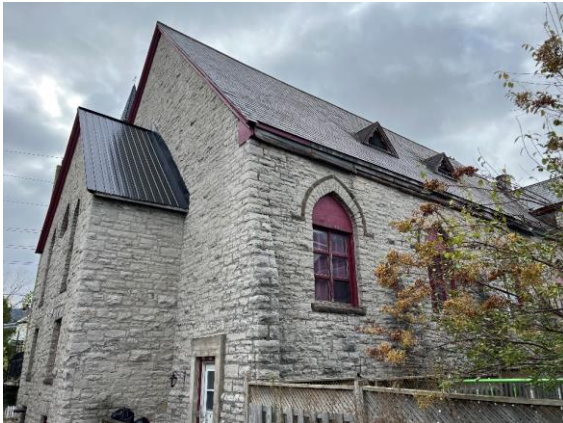
Photo 19: Missing Eavestroughs
