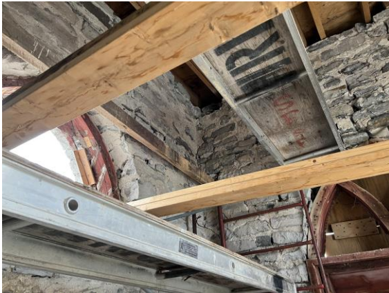
Photo 9: Interior Condition of Southeast Corner
