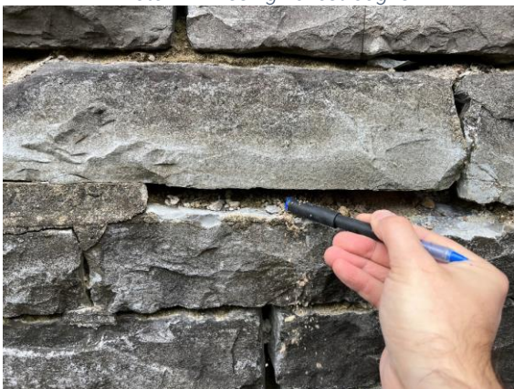
Photo 21: Joint being Raked with a Pen
