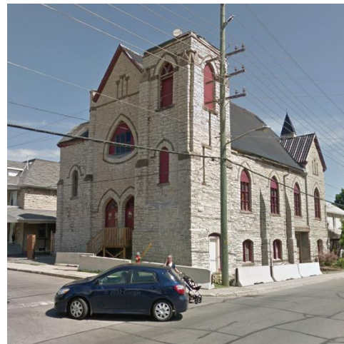
Figure 3: Another Partial Removal of Belltower (Google Street view 2016)
