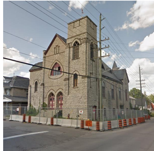
Figure 2: Belltower Partially Removed (Google Street view 2012)
