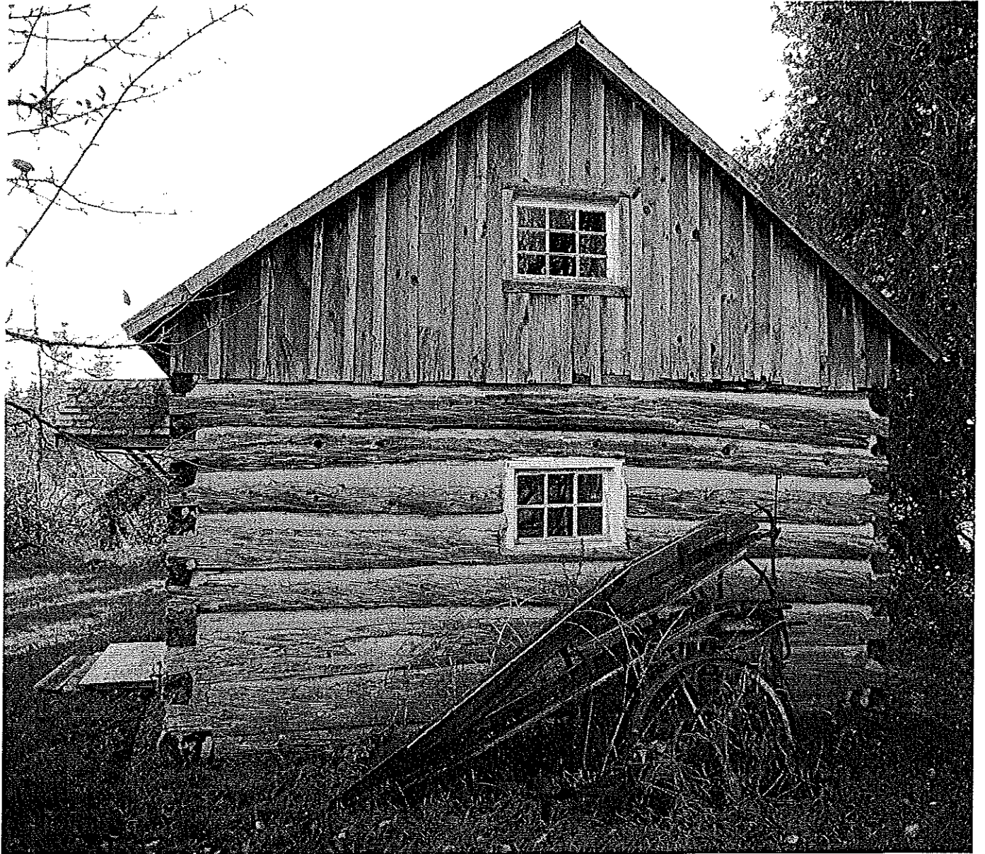
Photograph 2 (east gable end)
