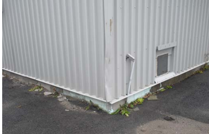
Photo 6: Well 5 - Cracked paving
