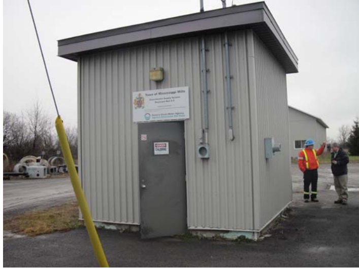
Photo 10: Well 5 - Redundant hydro meter base and conduits
