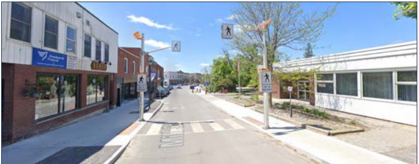
Figure 16: Mill Street PXO facing west (Source: Google)
