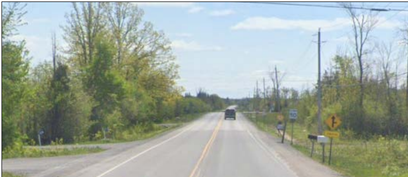
Figure 37: Appleton Side Road at Ottawa Street facing south (Source: Google)
