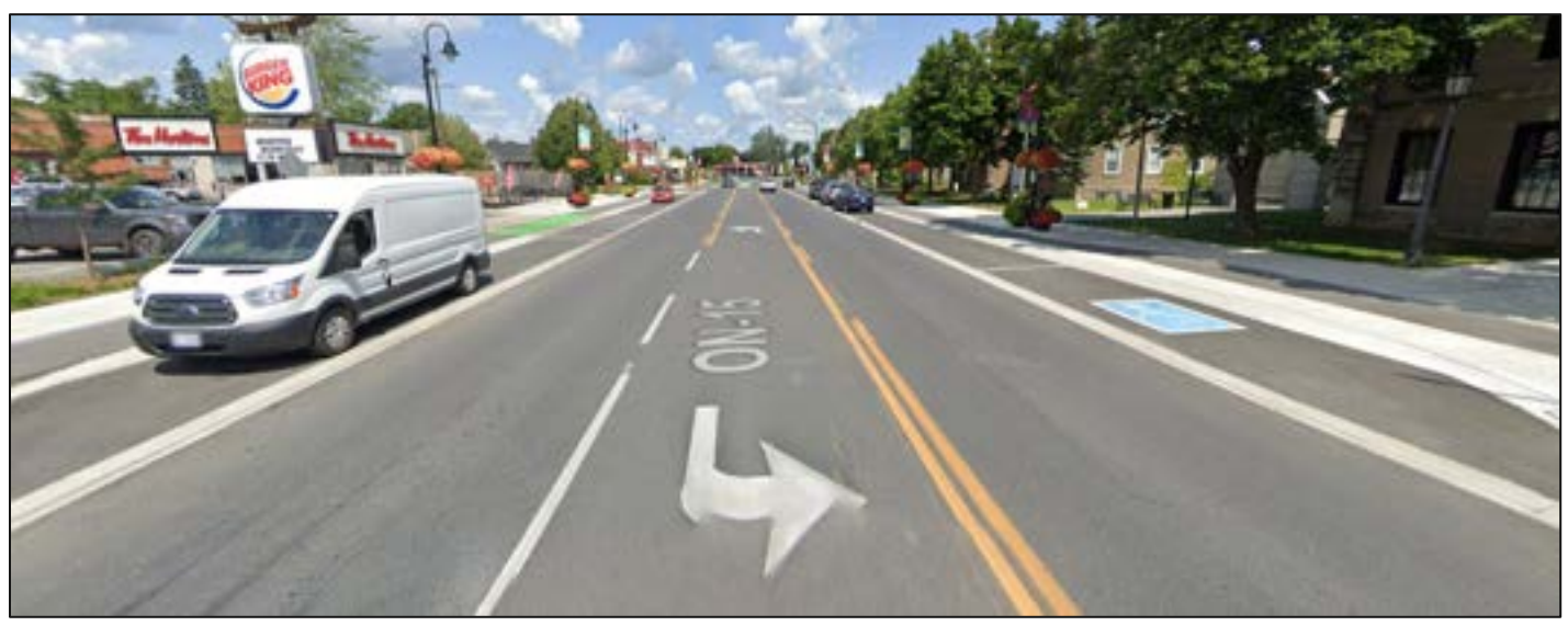
Figure 10: Example of Accessible Parking Bays, Beckwith Street, Smiths Falls (Google Maps, 2023)
