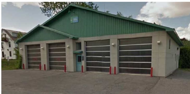
Figure 7: Mississippi Mills Station 2, Pakenham
