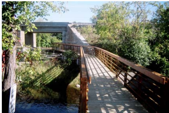
Riverwalk Bridge continuing under Railway Trestle
