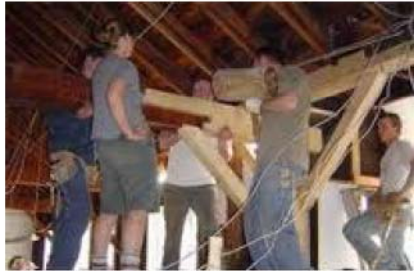
Restoration of the Almonte Agricultural Hall, 2004
