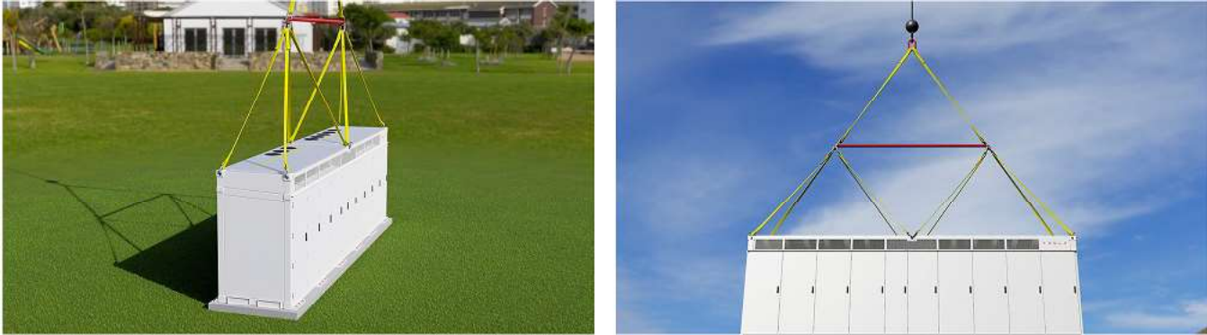
Figure 5. Lifting Using Straps and a Spreader Bar
