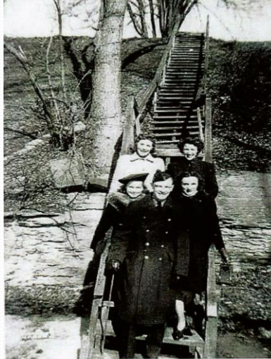
Mill Workers Walkway (aka Bank Street), connecting Union Street to Rosamond Mill on Coleman Island.
